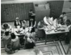
Ryerson Interiors, First Floor (109-9.5-1.1)
