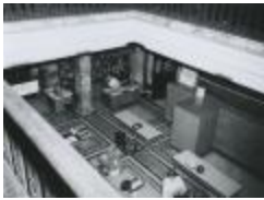
Ryerson Interiors, First Floor (109-9.5-2.4)
