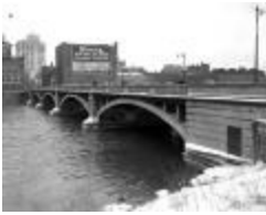
Pearl Street bridge (125-h001990_009)
