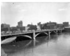
Fulton Street bridge (125-h001990_004)
