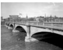
Bridge Street bridge (125-h001990_006)
