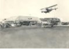
Kent County Airport (54-16-13.3271)
