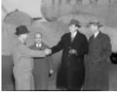
Airport, Works Progress Administration inspectors (125-h000161_002)
