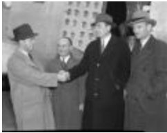
Airport, Works Progress Administration inspectors (125-h000161_001)
