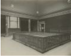
Ryerson Interiors, Second Floor (109-9.5-10)
