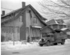
Allied Roofing (125-h000239_001)
