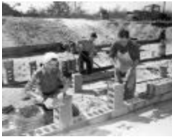
Abel building own house at 9105 Vergennes (125-h000009_003)
