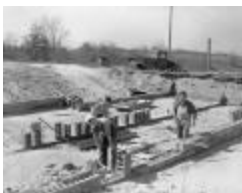
Abel building own house at 9105 Vergennes (125-h000009_002)
