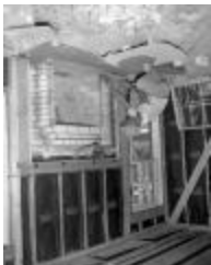
Albert Builders, new house (125-h000179_003)
