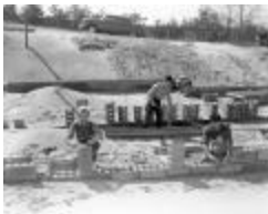
Abel building own house at 9105 Vergennes (125-h000009_001)
