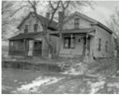
Housing Survey, bad houses (125-h008683_004)
