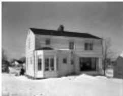
Radiant Heating & Supply Co. (125-c031545_004)
