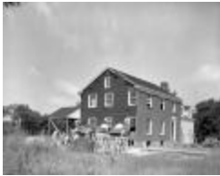
Albert Builders, new house (125-h000179_004)
