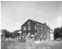
Albert Builders, new house (125-h000179_001)
