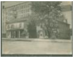
Division Street view (18-2-1.104.1861)
