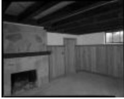
Recreation Room paneling (125-o1434_002)
