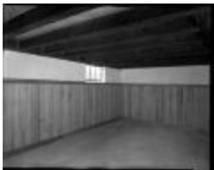
Recreation Room paneling (125-o1434_003)
