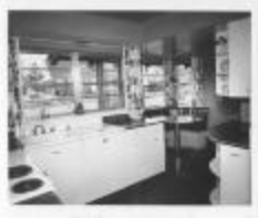
1338 Parkhurst Ave NW, interior (482-001-006_003)
