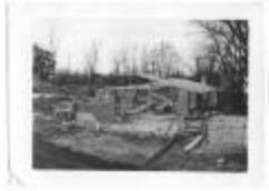
77 Lakeview SE Construction (482-001-014_001)
