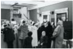
Ryerson Interiors, First Floor (109-9.5-5.5)
