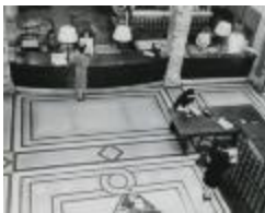
Ryerson Interiors, First Floor (109-9-31.2)
