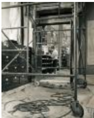
Ryerson Interiors, Second Floor (109-9.5-15.1)
