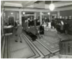
Ryerson Interiors, First Floor (109-9-31.4)
