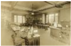
Ryerson Interiors, First Floor (109-9-16.3786)
