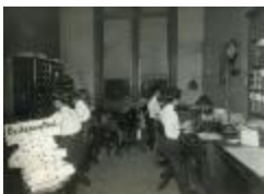
Ryerson Interiors, First Floor, Secretary's Office (109-9-20.36)
