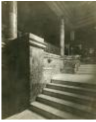
Ryerson Interiors, Stairway (109-9.5-7.1754)
