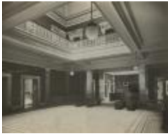
Ryerson Interiors, First Floor, Lobby (109-9-30.1757)
