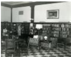
Ryerson Interiors, First Floor, Browsing Room (109-9-22.1)
