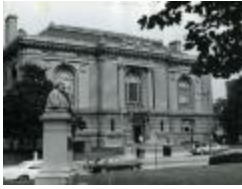
Ryerson Building Exterior (109-9-8)
