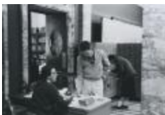
Ryerson Interiors, First Floor (109-9.5-5.4)
