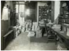
Ryerson Interiors, Basement Rooms (109-9-13.23)
