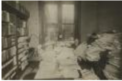
Ryerson Interiors, First Floor, Librarian's Office (109-9-21.060)
