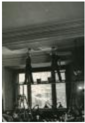
W.P.A. Cleaning Project (109-9.5-14.1)
