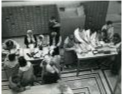
Ryerson Interiors, First Floor (109-9.5-1.1)
