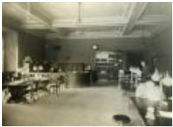
Ryerson Interiors, First Floor (109-9-16.2601)
