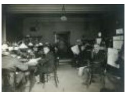
Ryerson Interiors, First Floor (109-9-17.4)
