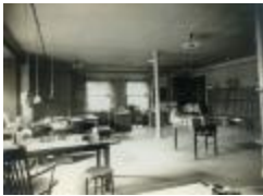
Ryerson Interiors, Basement Rooms (109-9-13.28)
