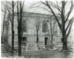
Ryerson Building Construction (109-9-4.25)
