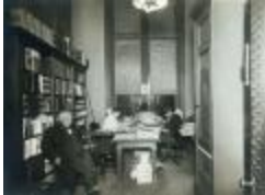
Ryerson Interiors, First Floor, Librarian's Office (109-9-21.24)
