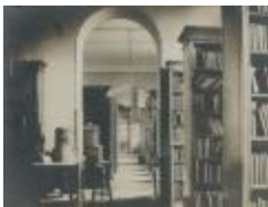
City Hall Library, corridor (109-9-1.15)
