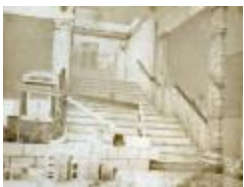
Ryerson Interiors, Stairway (109-9.5-7.2)
