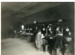
Ryerson Interiors, First Floor (109-9-16.3791)
