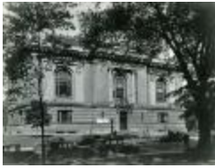
Ryerson Building Exterior (109-9-6.2)
