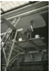
W.P.A. Cleaning Project (109-9.5-14.3785)
