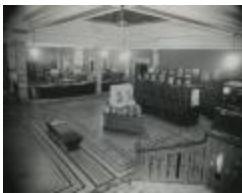
Ryerson Interiors, First Floor (109-9-31.3)
