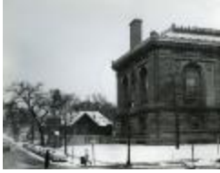
Ryerson Building Exterior (109-9-7.3895)
