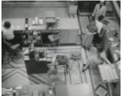
Ryerson Interiors, First Floor (109-9.5-1.2)
