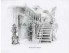
LLC Building Interior 1901 (275-037-014.1)
