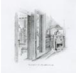
LLC Building Interior 1901 (275-037-014.2)
