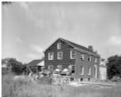
Albert Builders, new house (125-h000179_004)
