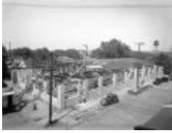
Building Construction (125-r36613_001)
