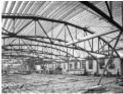
Building Construction (125-r36614_001)
