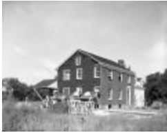
Albert Builders, new house (125-h000179_001)
