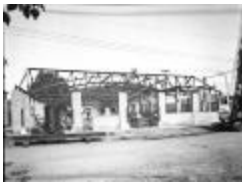
Building Construction (125-r36615_001)
