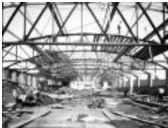
Building Construction (125-r36618_001)
