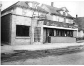
Bronkema Builders Office (125-h002026_001)
