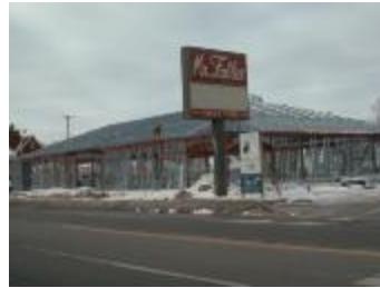
Construction of West Leonard Branch (109-127-GNW2002-01-05-DSC00005)
