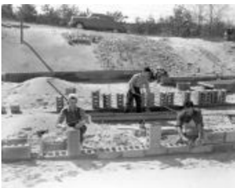
Abel building own house at 9105 Vergennes (125-h000009_001)
