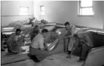
Wengers Bowling Alley Construction (125-o1016_001)
