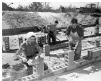
Abel building own house at 9105 Vergennes (125-h000009_003)
