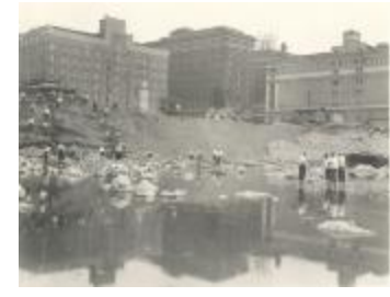
Welsh Auditorium Construction (43-2-2.422)
