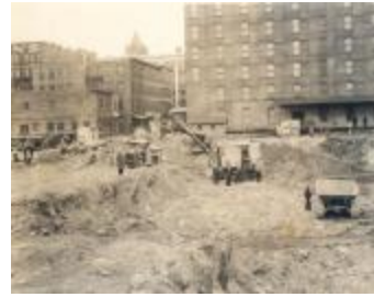
Welsh Auditorium Construction (43-2-2.420)
