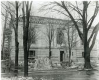
Ryerson Building Construction (109-9-4.25)
