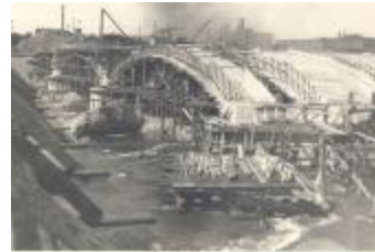
Construction of the Fulton Street Bridge (43-1-2.61A)
