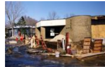
Yankee Clipper renovation (109-037-055_001)
