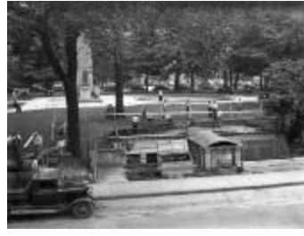
Construction in Veterans Park (125-r35225_001)
