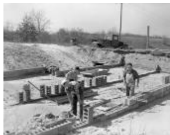
Abel building own house at 9105 Vergennes (125-h000009_002)
