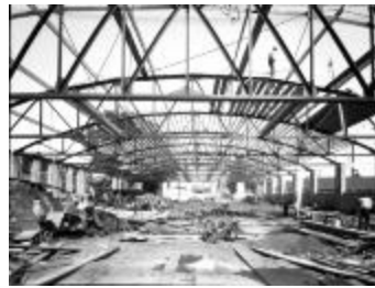
Building Construction (125-r36618_001)
