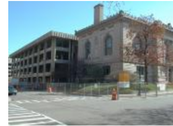
Main branch, 2000 renovation (109-digital_grm9)
