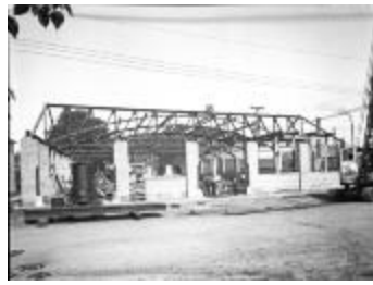
Building Construction (125-r36615_001)
