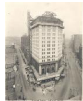
McKay Tower Construction (43-1-2.94)
