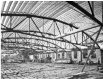
Building Construction (125-r36614_001)
