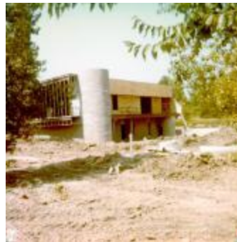
Yankee Clipper construction (109-026-040_002)
