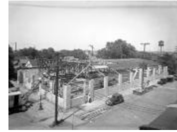
Building Construction (125-r36613_001)
