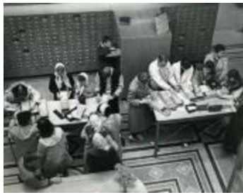
Ryerson Interiors, First Floor (109-9.5-1.1)
