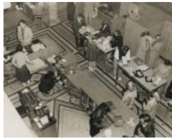
Ryerson Interiors, First Floor (109-9.5-1.3)
