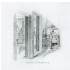
LLC Building Interior 1901 (275-037-014.2)
