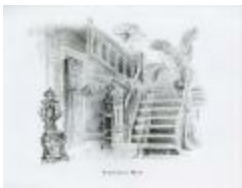
LLC Building Interior 1901 (275-037-014.1)
