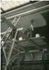
W.P.A. Cleaning Project (109-9.5-14.3785)
