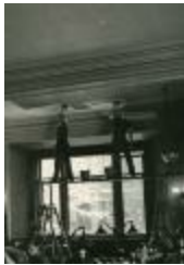
W.P.A. Cleaning Project (109-9.5-14.1)
