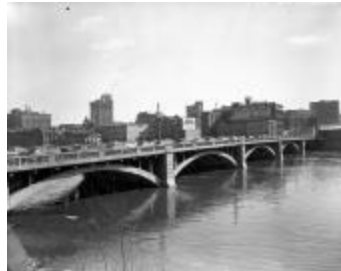
Fulton Street bridge (125-h001990_004)
