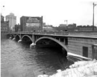
Pearl Street bridge (125-h001990_009)
