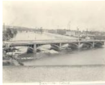
Fulton Street Bridge over the Grand River (43-1-2.59)
