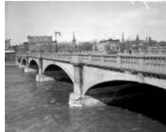
Bridge Street bridge (125-h001990_006)
