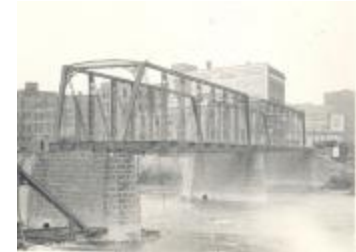
Fulton Street Bridge (43-1-2.66)
