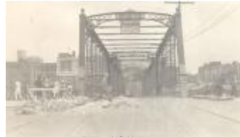
Fulton Street Old Iron Bridge (43-1-2.64)
