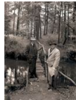
Foot bridge (125-r35304_001)
